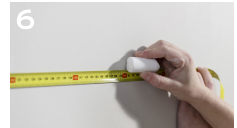
6 Loosely measure and mark your horizontal and vertical lines with chalk.
